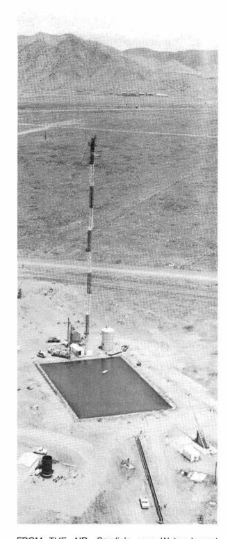
FROM THE AIR, Sandia's new Water Impact Target resembles a swimming pool with the world's tallest diving tower. The facility allows precision control and full instrumentation coverage during high impact tests of large test units onto the surface of the 50-foot-deep pool.
